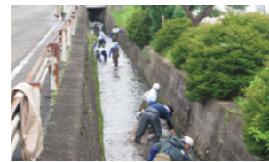
Volunteer river cleanup work in the Sakura area
